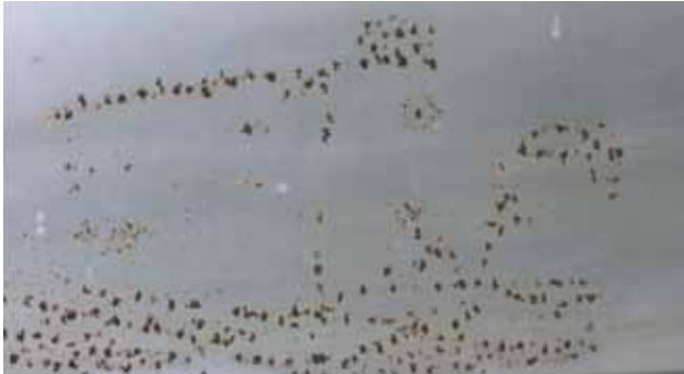
Chlorine corrodes stainless steel
