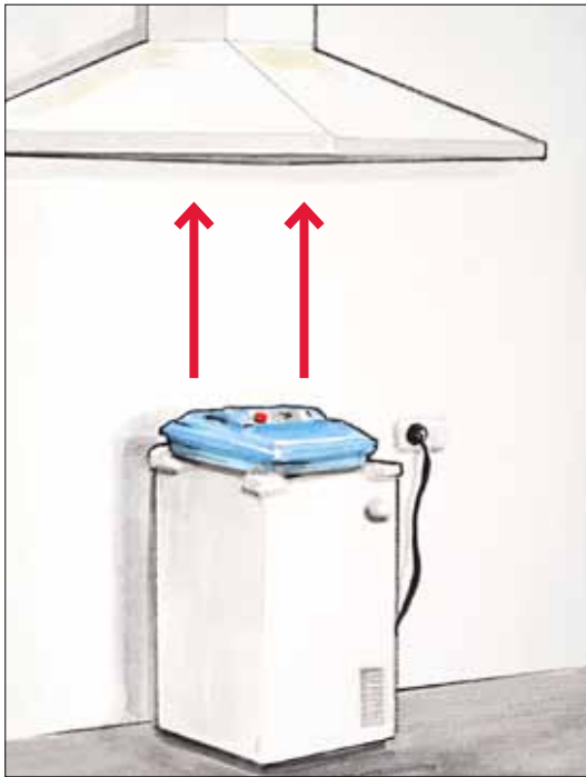
Thimble exhaust over a steam pressure sterilizer
